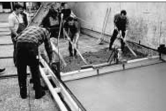
Fig. 1: Concreting preparations on the Meiereihof
