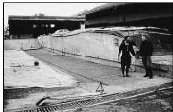
Fig. 2: Post-concreting treatment through covering
