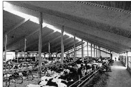
Fig. 2: Exterior feed troughs such as here on the Gaidetzka unit enable a compact design even with large herds
