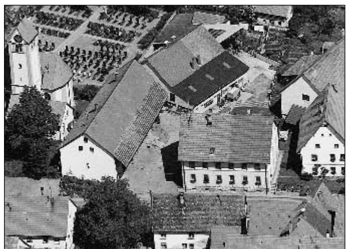
Fig. 5: Alongside the church, the home of the Hölz family. In the old farm buildings only the farrowing area has been extended
