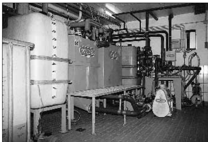
Fig 2: Feed centre including acidification facility at a modern weaner production unit
