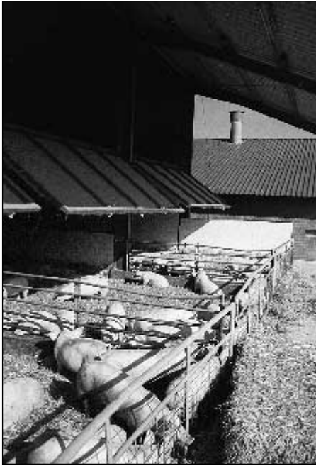
Fig. 2: Open-front house with moveable front covers for feeding pigs (Photos: W. Achilles)
