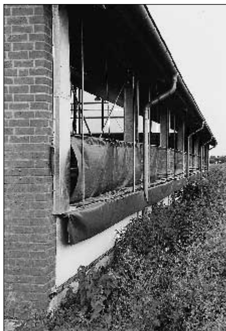
Fig. 2: Adjustable roller blinds allow a higher air exchange rate (photos: W. Achilles)
