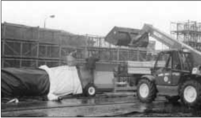
Fig 2: Filling the foil hose fermenter
