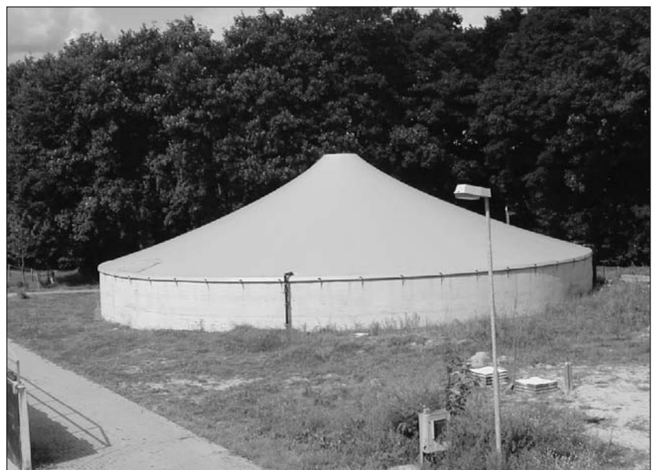
Fig. 1: Slurry container made of reinforced concrete with cover „tent“ type
