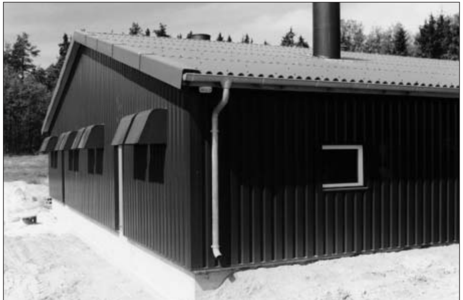
Fig. 2: At this pig fattening house cover trapezoidal corrugated sheets were used as facing (Photo: Laukien Comp., Kiel)
