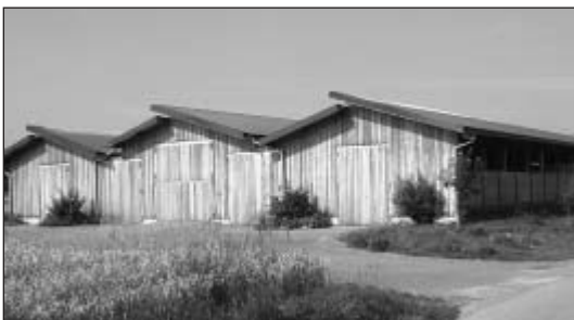
Fig. 2: The Sedlmair farm convinces with a practice oriented construction and a landscape-friendly building
