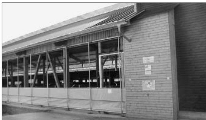
Fig. 4: Fresh air free ventilation through the side wall with roll-up covers
