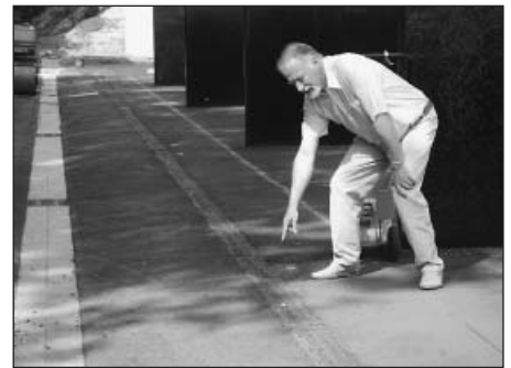
Fig. 2: Arrangement of concrete slit and drain trench
