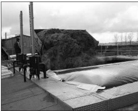
Fig. 3: Filling the two-level digester (source: Ratzka consulting engineers)
