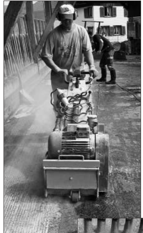
Fig. 1: Milling device, with continuously variable drives for lengthways grooving. Small picture: Combination of round and octagonal milling cutters
