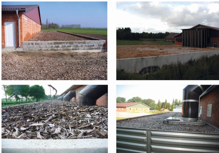
Figure 1: Single stage bio filters for odor reduction from animal houses (© J. Hahne)
